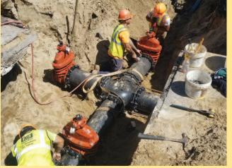
Work was recently completed to install a 12-inch cross-tee and valve-cluster to help ensure the Authority's ability to adjust system flow patterns during an emergency situation. A large excavation area was needed at the intersection of Bayview Avenue and Cedar Drive to connect the newly configured piping to the existing distribution system.
